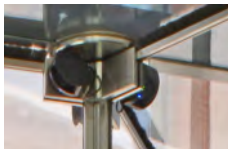
Top Hanger: It facilitates the rotation motion and is positioned at the top of rotating structure. This part has a unique design in terms of its dimension.
